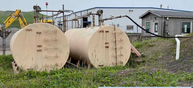
Upgrades are recommended to reduce the risk of spill during transfer of gasoline through existing flexible piping and single wall tankage.
